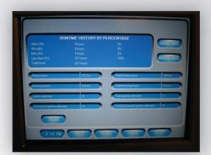
The Crest's 'best-in-class' modulation has helped cut fuel costs as the boiler has been operating at less than 25% modulation since installation.
