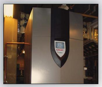
reset functionality, one of the many features offered with its exclusive SMART TOUCH<sup>™</sup> operating control. Since outdoor reset adjusts the heating system water temperature based on the outdoor air temperature, it allows for decreased fuel consumption and increased consistent comfort.
